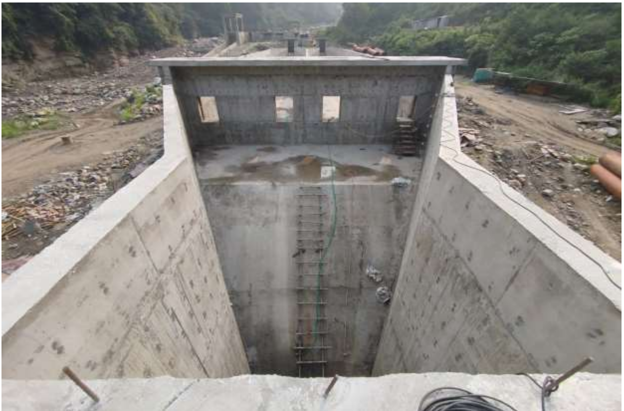
Figure 6: Forebay structure after completion.
