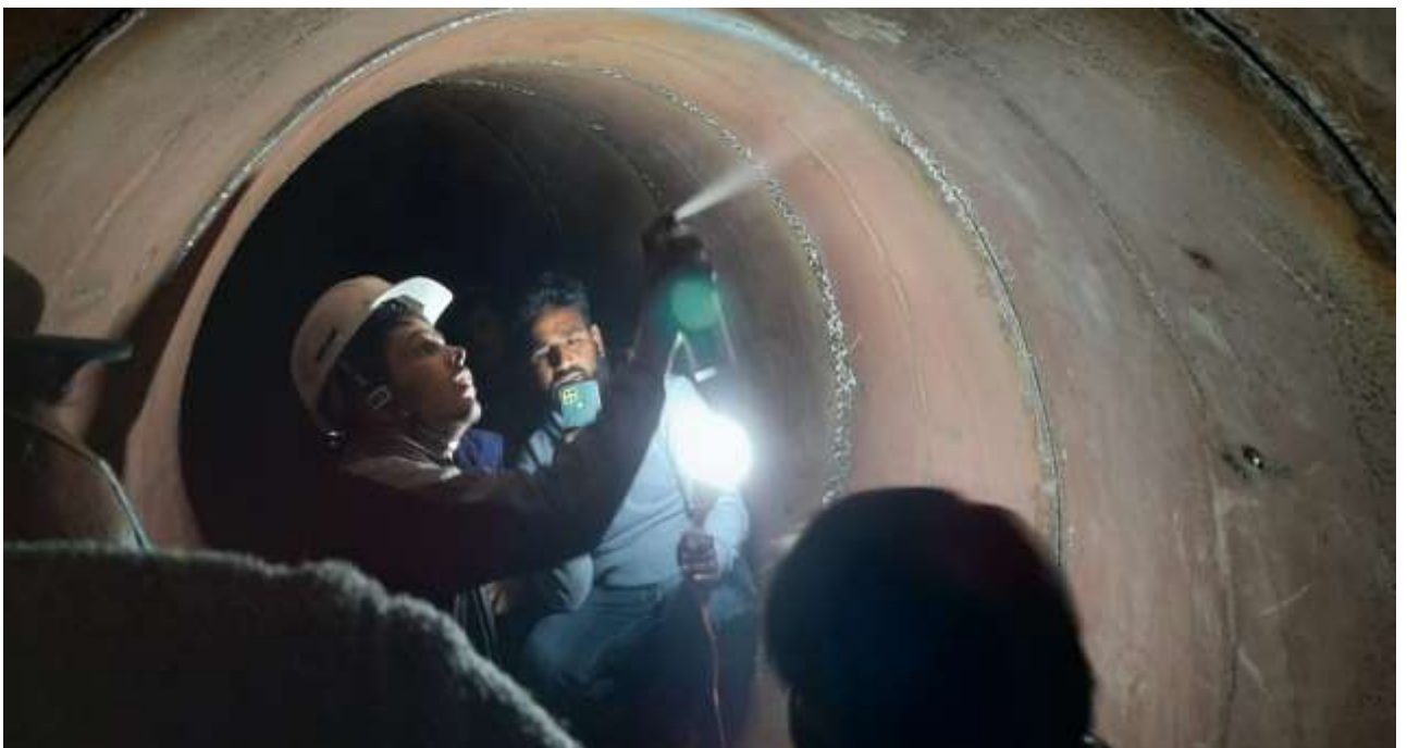
Figure 18: NDT test in pipe welding.
