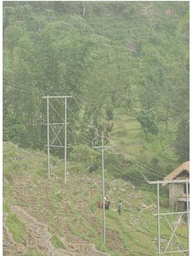
Figure 23: Pole and conductor installation in transmission line.
