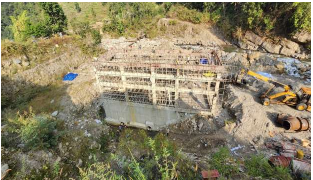
Figure 14: Overall Powerhouse Area.
