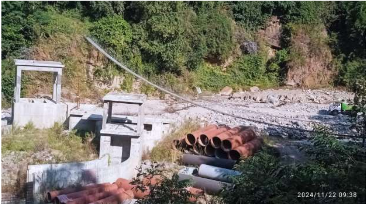
Figure 1: Headworks upstream side.
