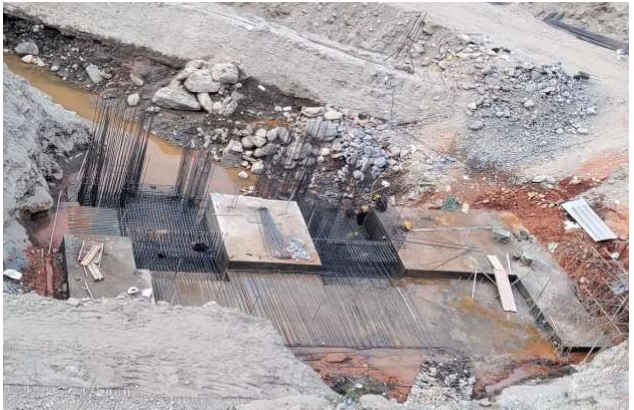
Figure 11: Rebar laying and concreting work at powerhouse draft tube and foundation.
