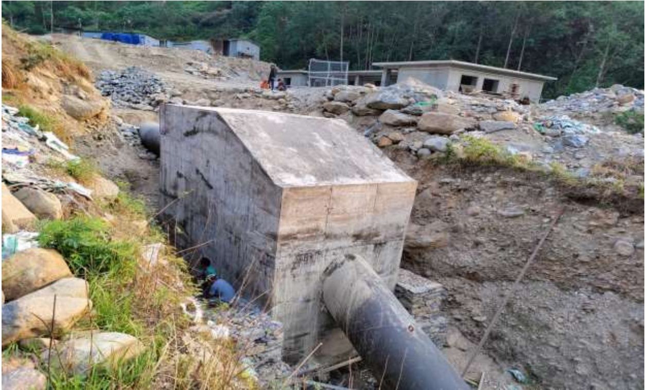
Figure 17: Installation bend and penstock pipe upstream of powerhouse.
