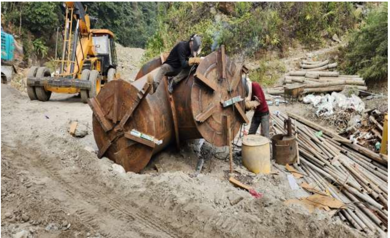
Figure 20: Bifurcation ready for pressure testing.
