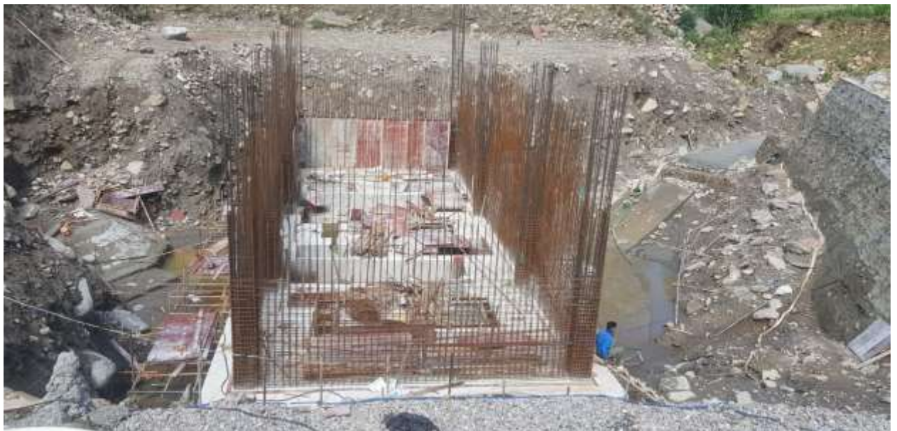
Figure 12: Powerhouse machine foundation.
