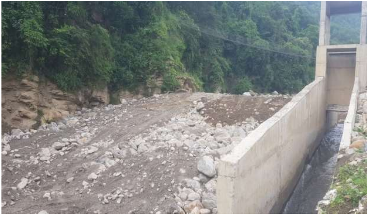
Figure 3: Weir after completion.
