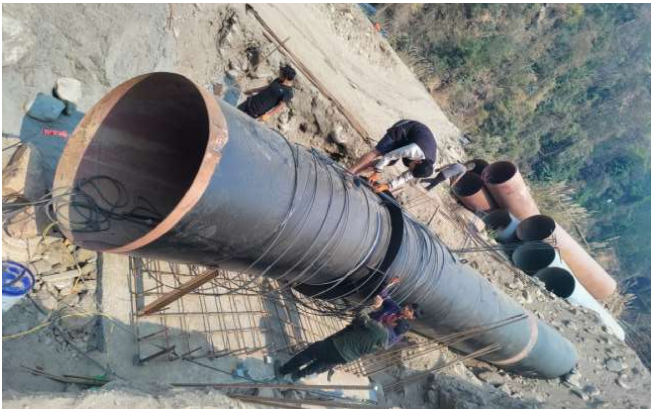
Figure 15: Pipe Installation and protection work.
