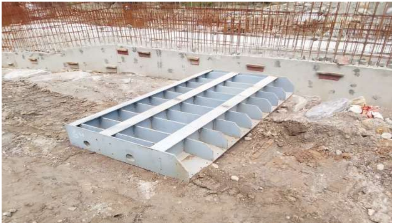
Figure 22: Intake gate leaf.
