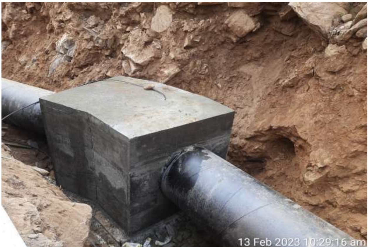
Figure 7: Syphon after final protection.
