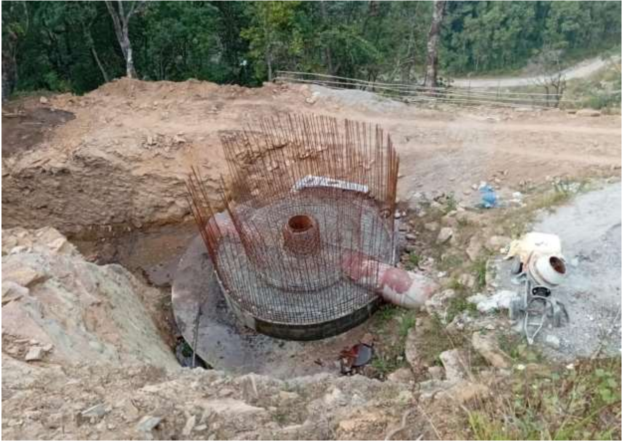
Figure 9: Surge tank Foundation and shear wall.
