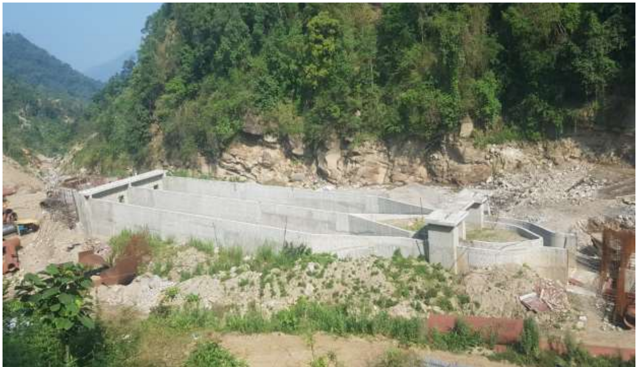
Figure 4: Settling basin after completion.
