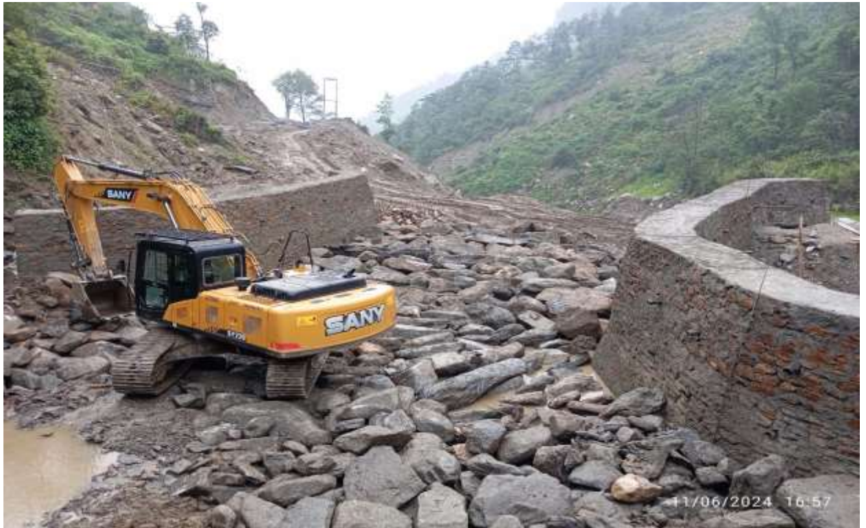
Figure 7: Syphon after final protection.
