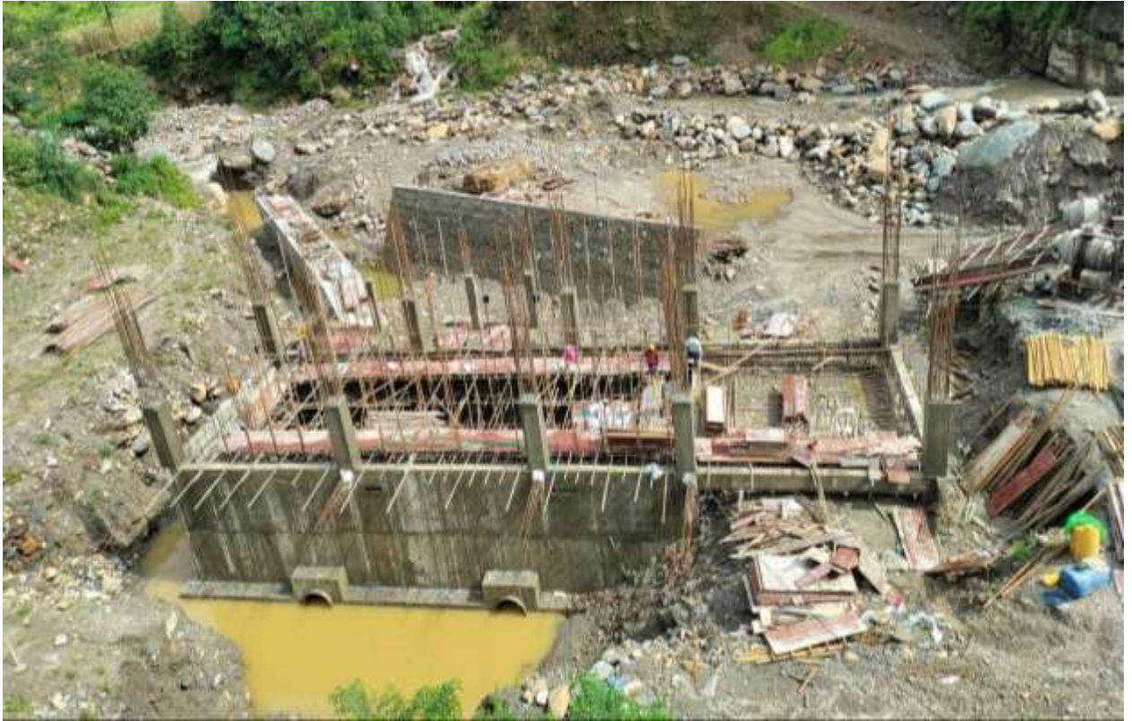
Figure 13: Powerhouse Shear wall and column above service bay level.
