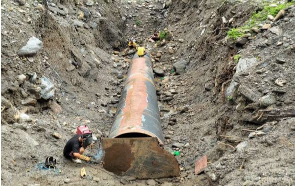
Figure 21: Penstock Pipe installation.
