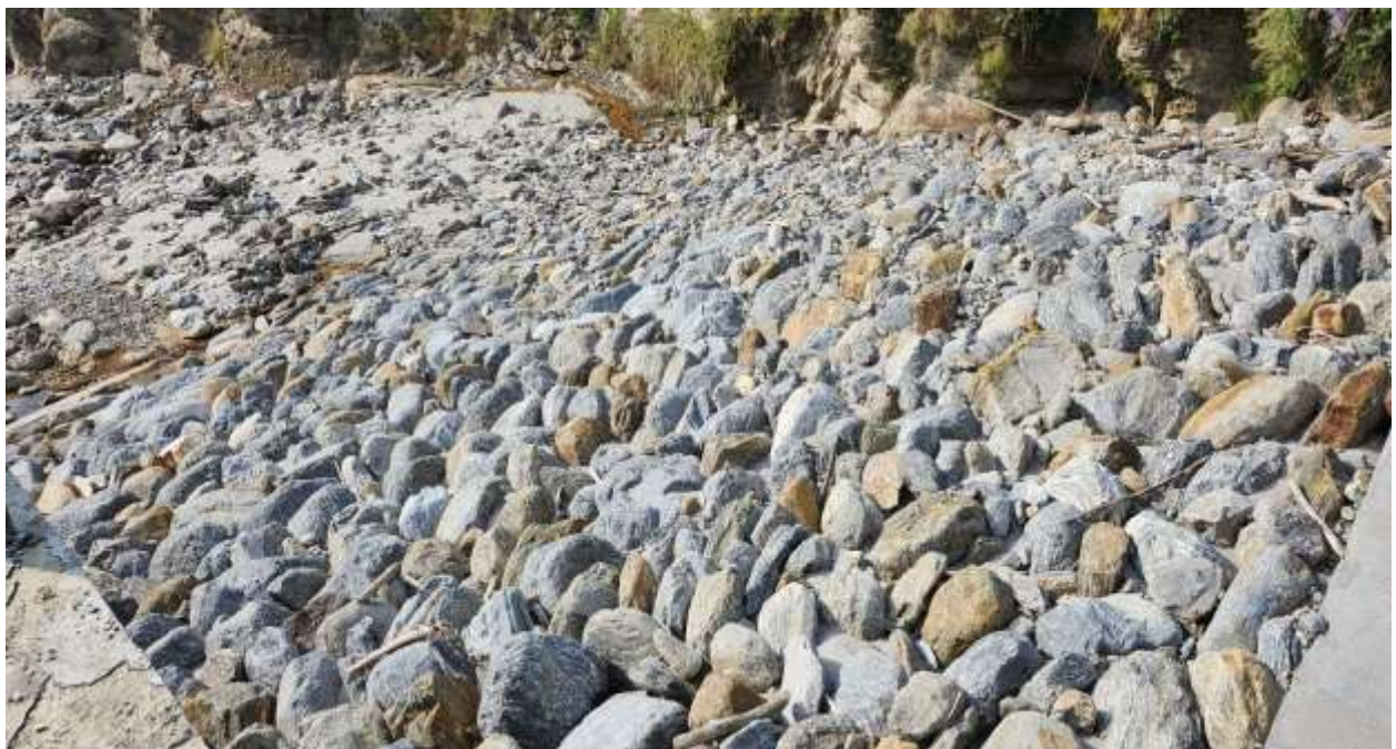
Figure 2: Weir and undersluice downstream side.
