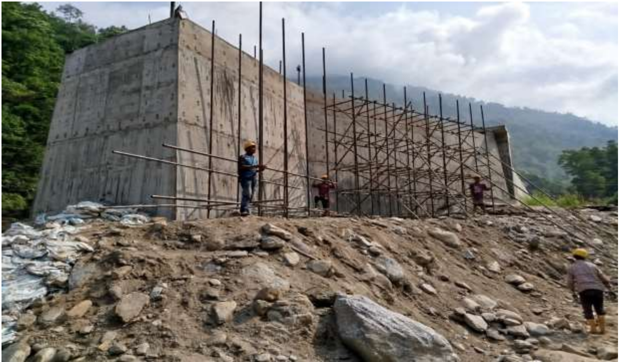
Figure 5: Forebay structure after completion.
