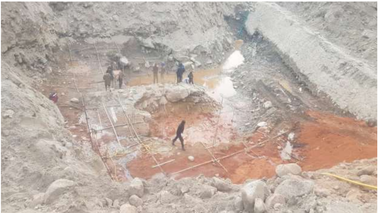
Figure 10: Installation of earthmat below powerhouse machine foundation.
